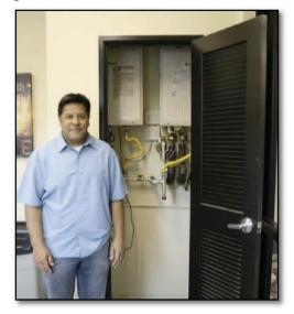
Greg Paulino with two of the condensing type tankless water heaters that were installed in the laundry rooms at Vintage Crossings. Paulino says he saved "between \$200 and \$300 on material costs for each of the two installs" by using PVC venting rather than stainless steel.
